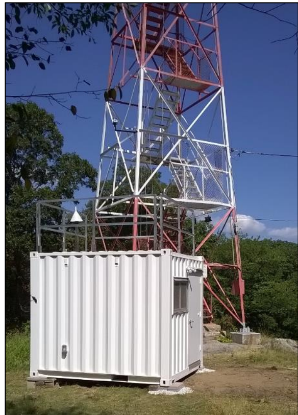
Figure 2-1 Ramapo Air Monitoring Station
